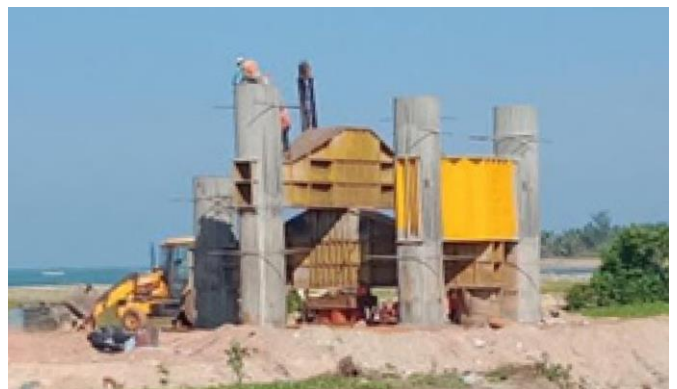
Fig: Ongoing works at Honnavar
