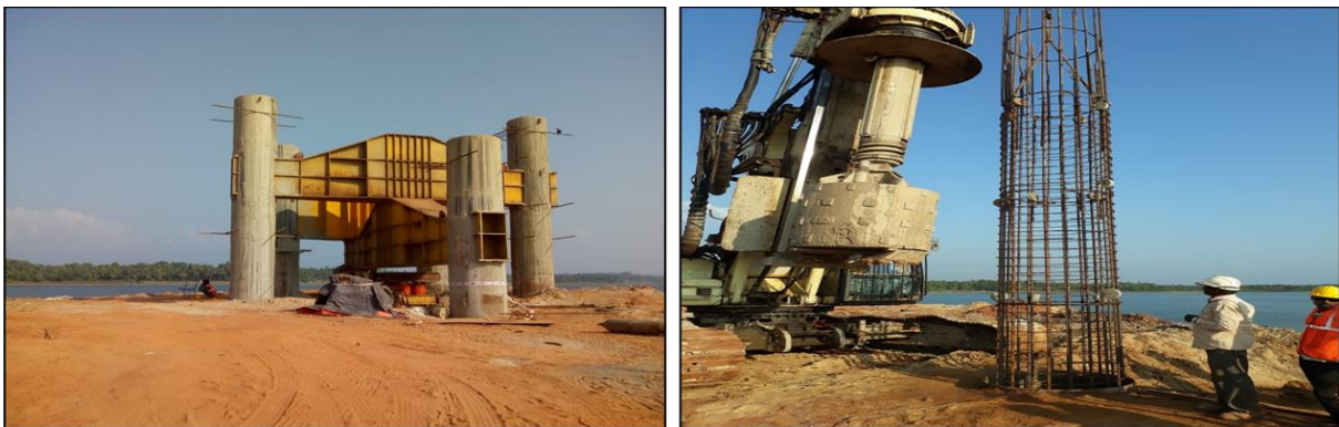
Figure 13: Images of work in progress at Honnavar Port
