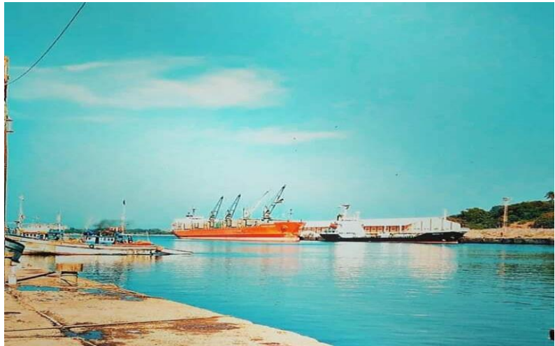
Figure 3: View of the Karwar Port
